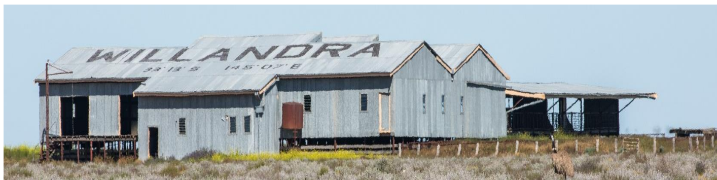
Figure 18: Willandra Shearing Shed, Carrathool LGA. Photo credit: Carrathool Shire Council.
