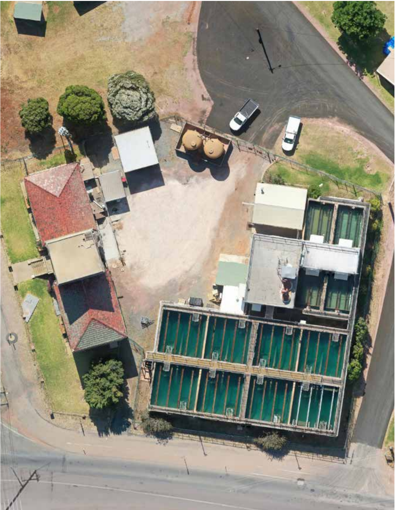
Overhead Water Filtration Plant
