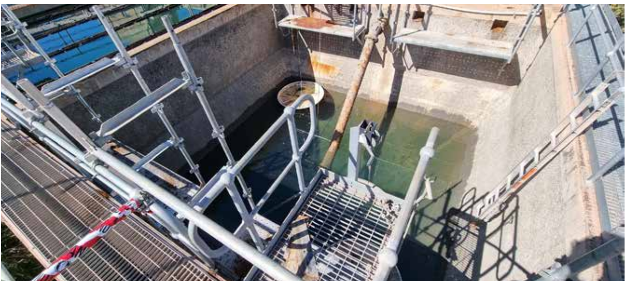
Launder replacement at the Leeton Water Treatment Plant
