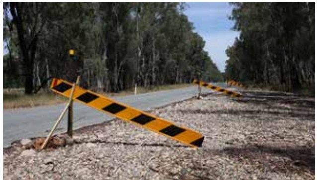
From the top: New bus shelter in Whitton Completed maintenance works on Wade Avenue Madonna Place footpath renewal Rehabilitation Works on Euroley Road
