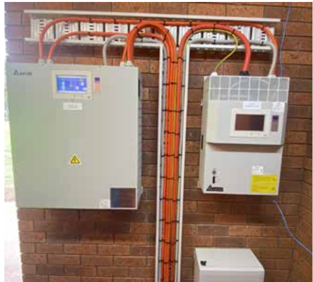
Electrical Upgrades at the Leeton Sewage Treatment Plant
