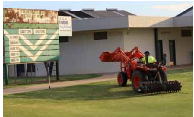
Leeton No 1 Oval Rehabilitation Works
