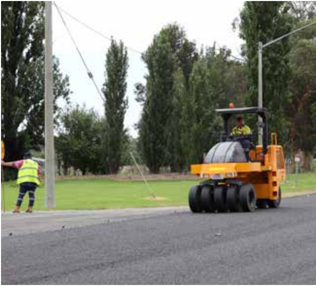
Brobenah Road Resealing
