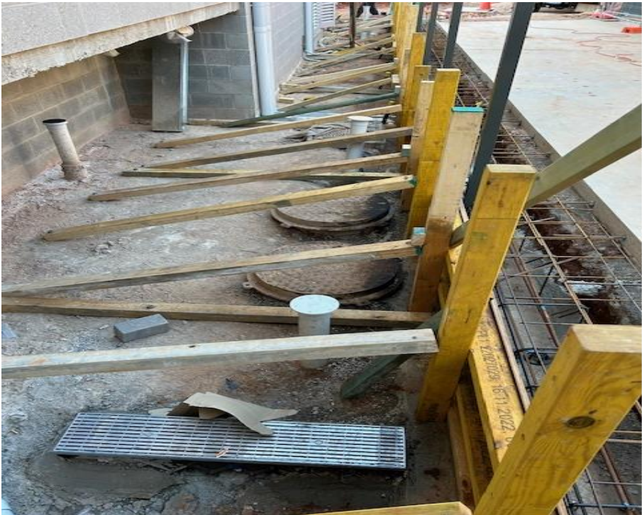
Photo: Rear disabled egress
