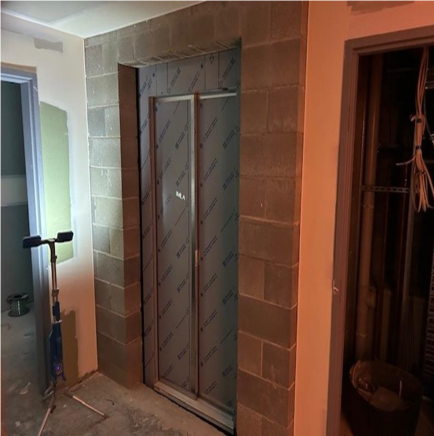
Photo: Completed lift installed.
