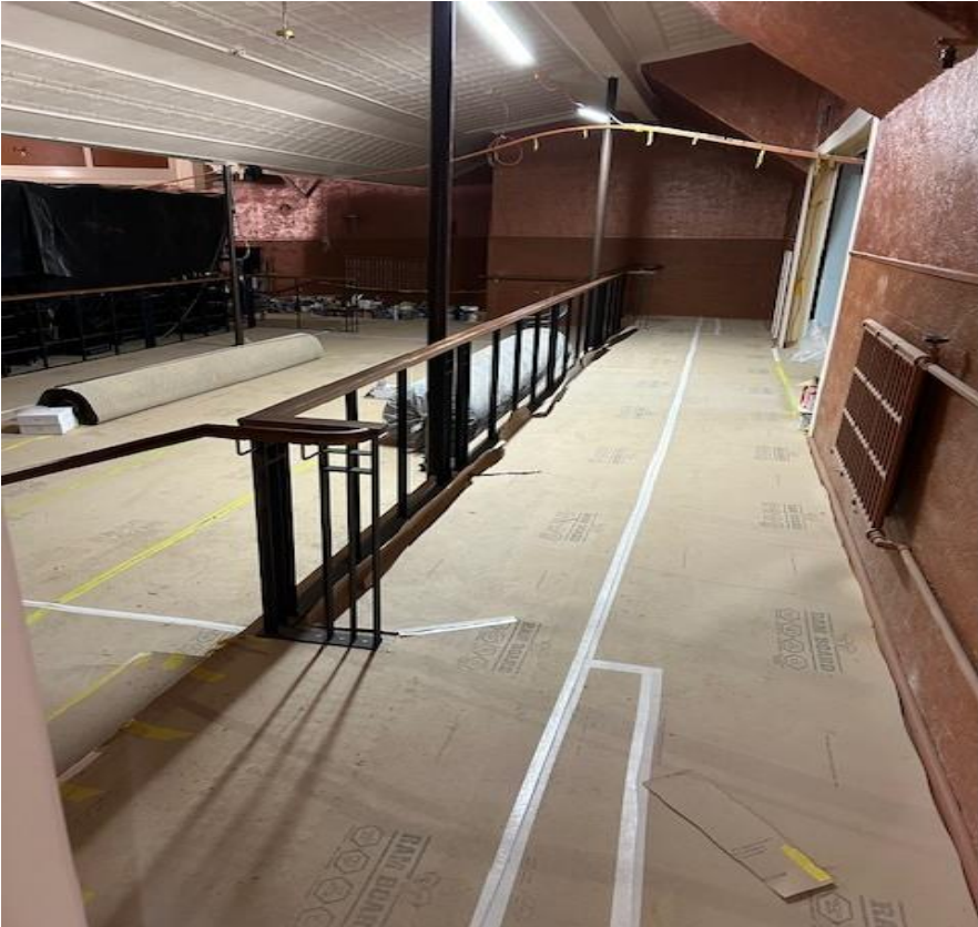
Photo: Completed balustrades. (Protective covering over new flooring)
