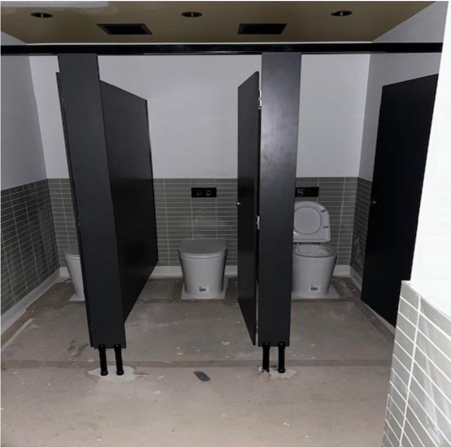
Photo: Completed amenities. (Protective covering over new flooring)
