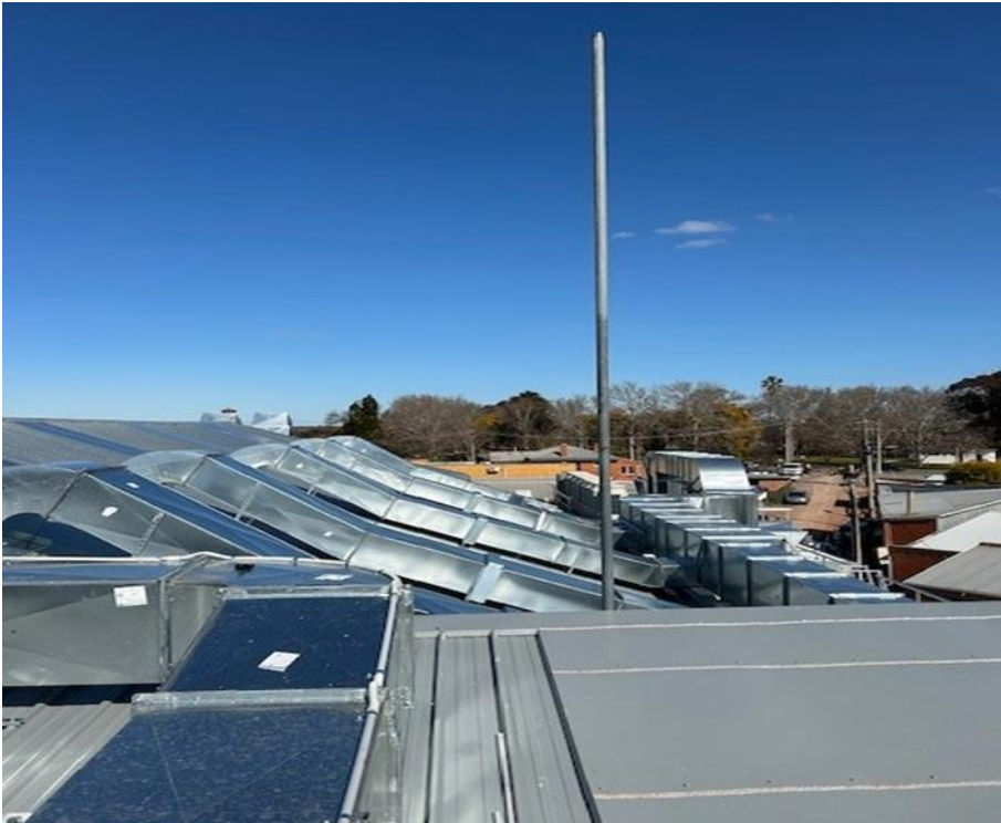
Photo: Completed mechanical duct work.
