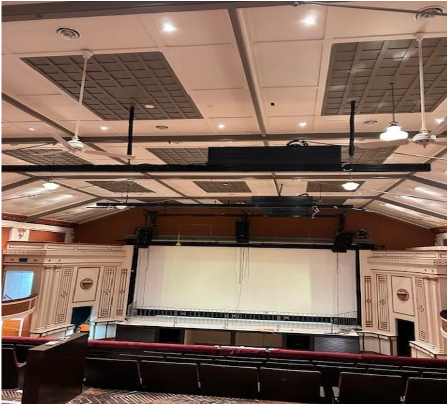
Photo: New lighting bars.
