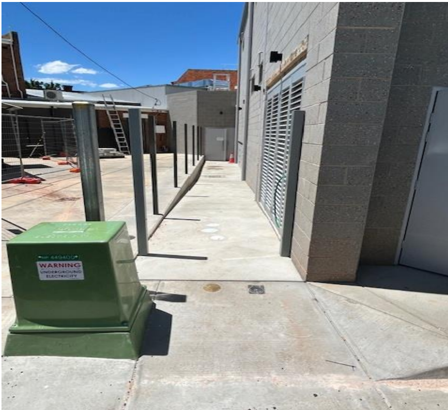
Photo: Emergency egress to Roxy Lane.
