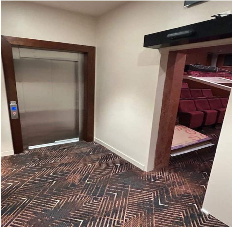
Photo: Completed lift lobby.
