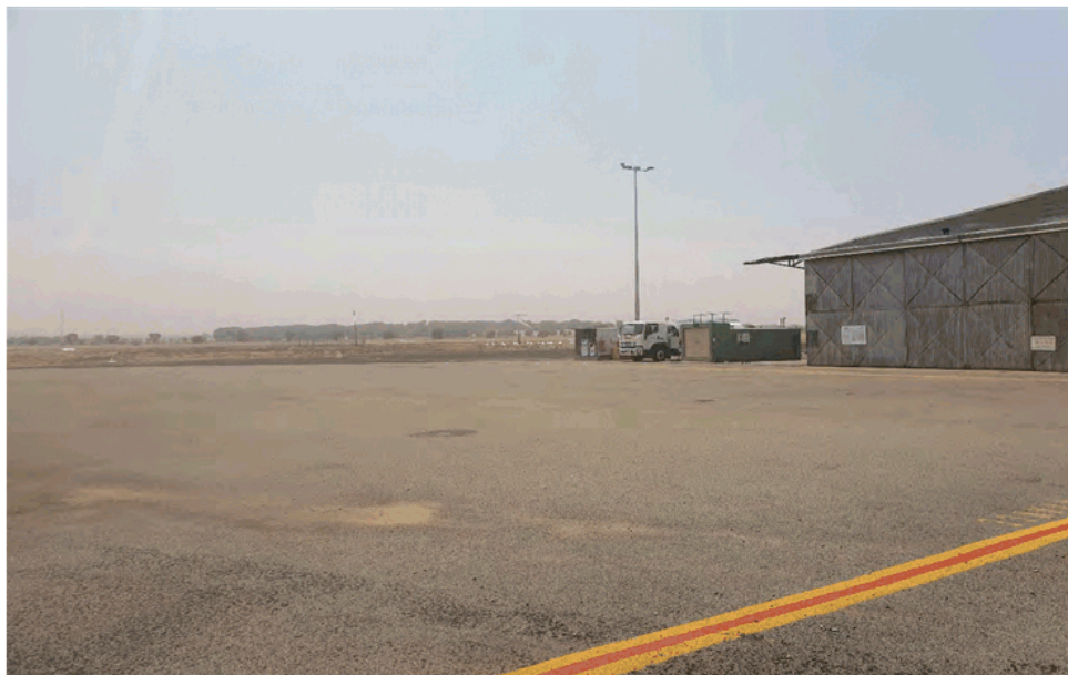
Fig 1 – Bellman Hangar as viewed from the Narrandera Terminal Building
