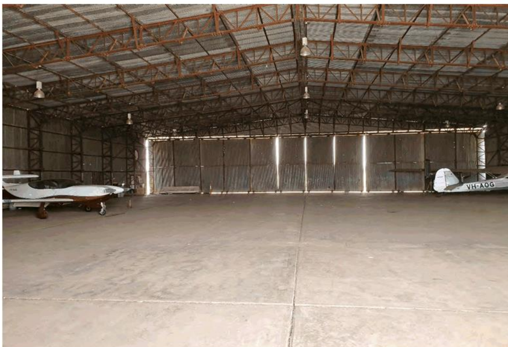
Fig 6 – Inside picture of the Bellman Hangar
