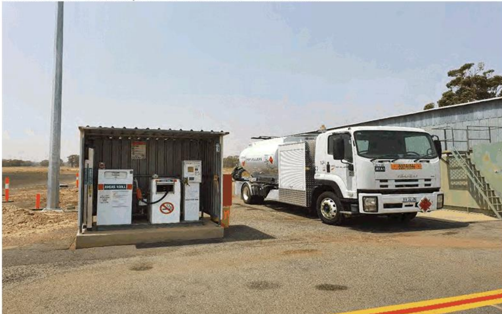
Fig 7 – The Refueling area at Narrandera Airport
