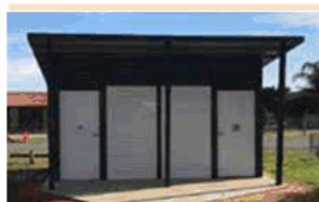
Above: Yanco's McCaughey Park benefitted from the construction of a new toilet facility with full disability access
