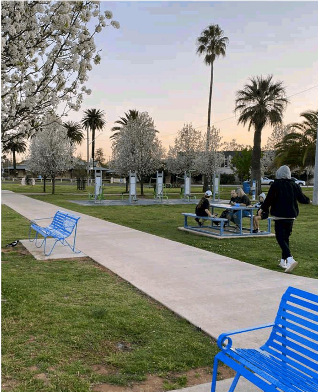
Council installed a new concrete path in Rotary Park, Leeton, to enable residents and visitors to skirt around the extended skate park
